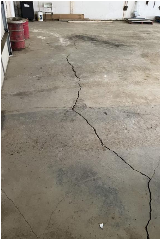
Cracks in floor
