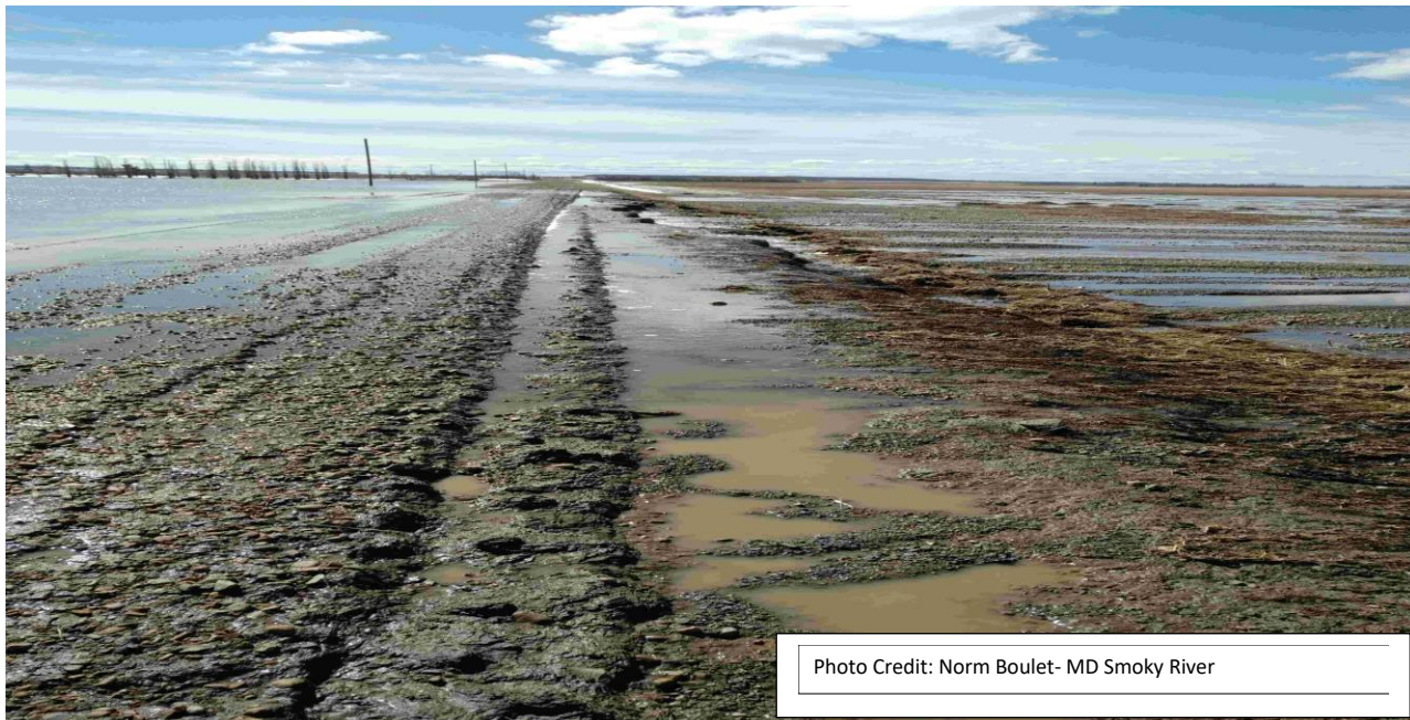
Picture 3: Road wash out due to field floods. No trees in sights
