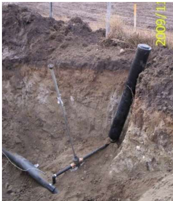
Photo 1: Automatic air release valve, before backfilling
