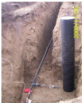
Photo 3: Meter vault installation prior to backfill
