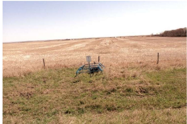
Photo 2: Manual air release hydrant
