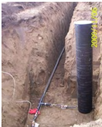
Photo 3: Meter vault installation prior to backfill
