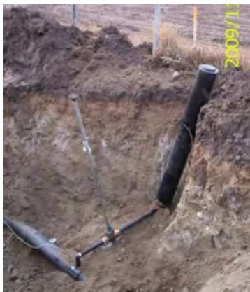
Photo 1: Automatic air release valve, before backfilling
