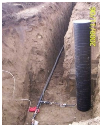
Photo 3: Meter vault installation prior to backfill
