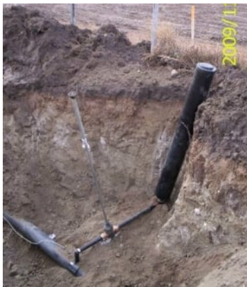
Photo 1: Automatic air release valve, before backfilling
